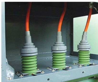
Installed Capacitive Couplers
