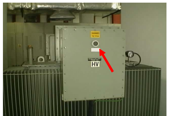
Transformer Terminations as seen thru HVIR Window
