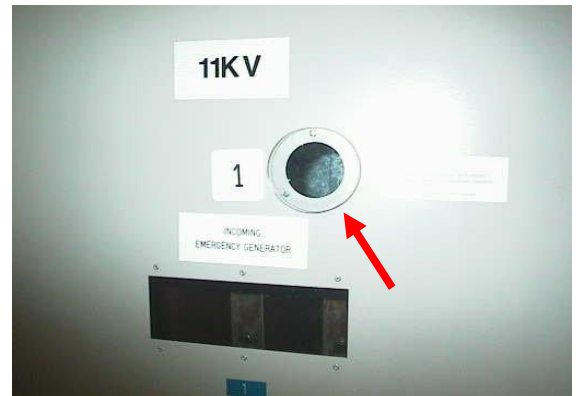
Busbar Terminations of a Switchgear as seen thru the HVIR Window
